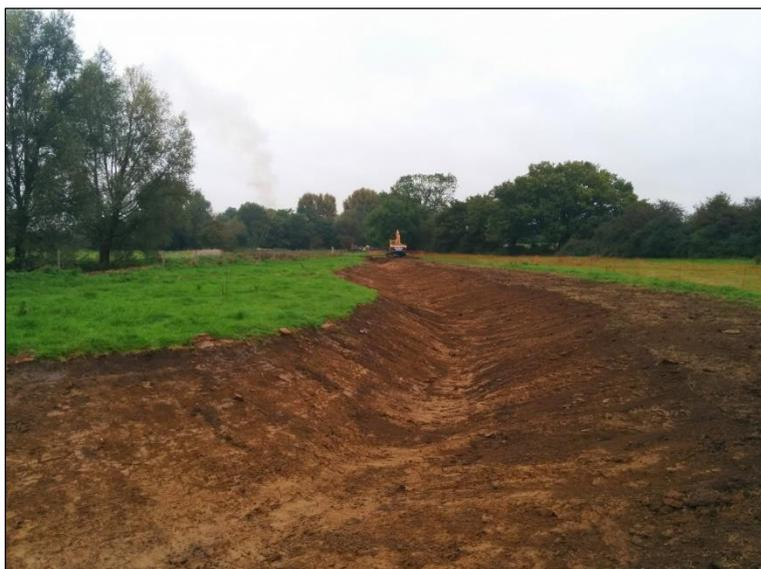
**Plate A1.6** Example of what construction of a back channel looks like.
