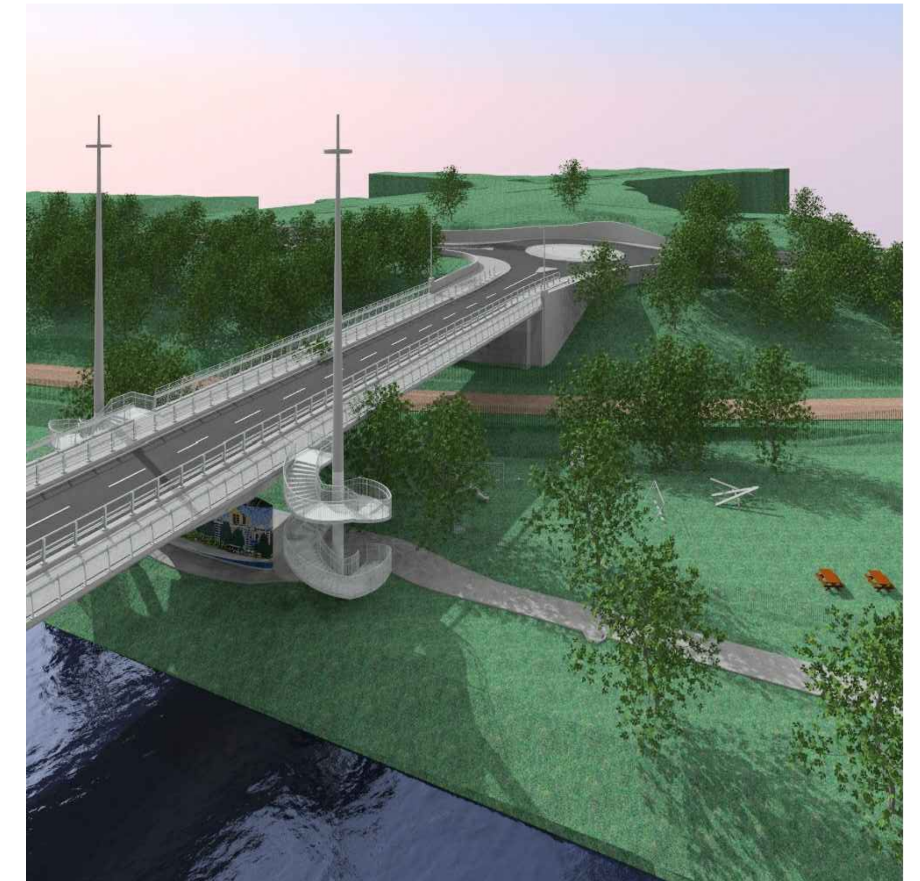
RIVER SLANEY BRIDGE AERIAL VIEW LOOKING WEST
