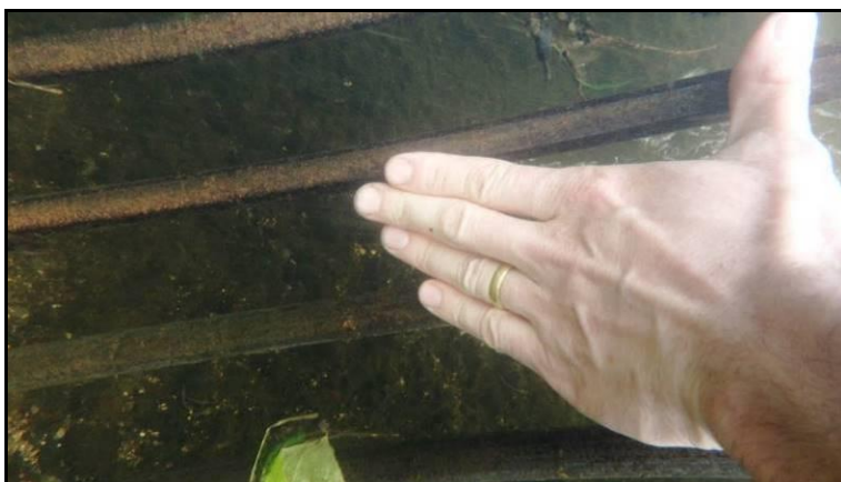
Plate 18: The spacing between the bars on the Clohamon hydro-scheme tailrace fish screen are in the order of 35mm. It is considered that River Lampreys could easily swim through this screen.
