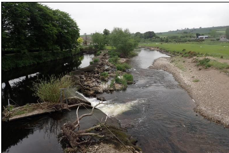
Plate 47: Clohamon weir on the 26 th May 2016. This is a major fish migration barrier.
