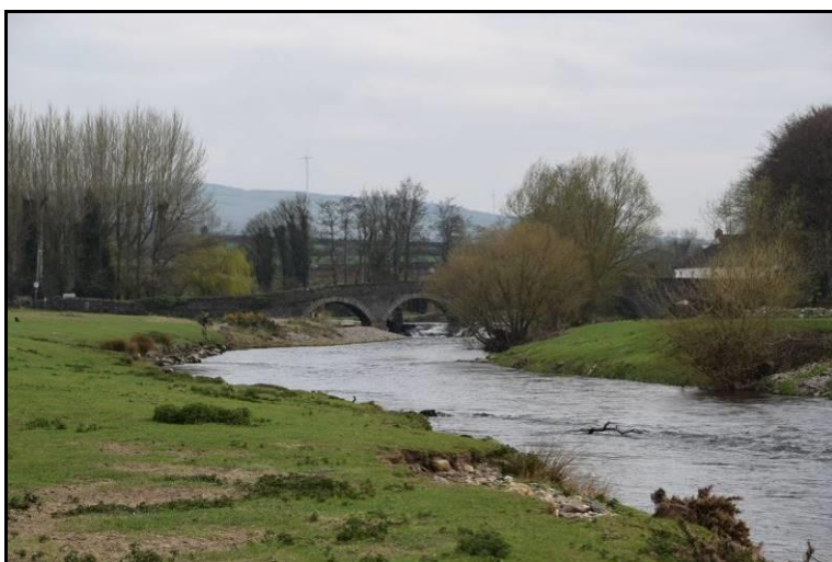
Plate 14: Stretch of the Slaney downstream of Clohamon Weir. This stretch of the river is depleted due to the operation of a small hydroelectric scheme at the left side of the channel.
