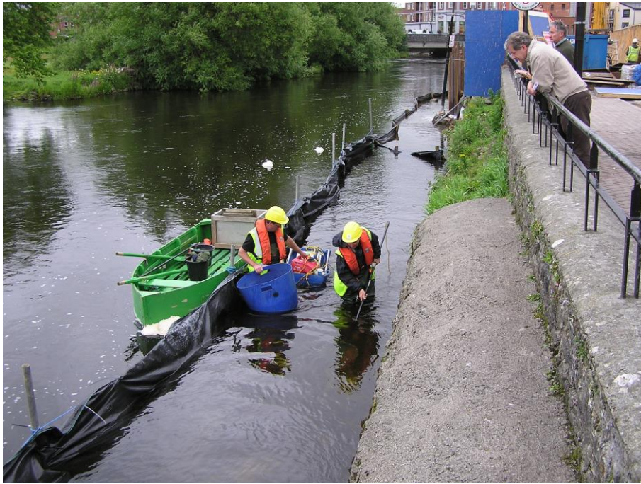
Plate 3 Fish translocation works on the Ennis Flood Scheme (Ecofact).
