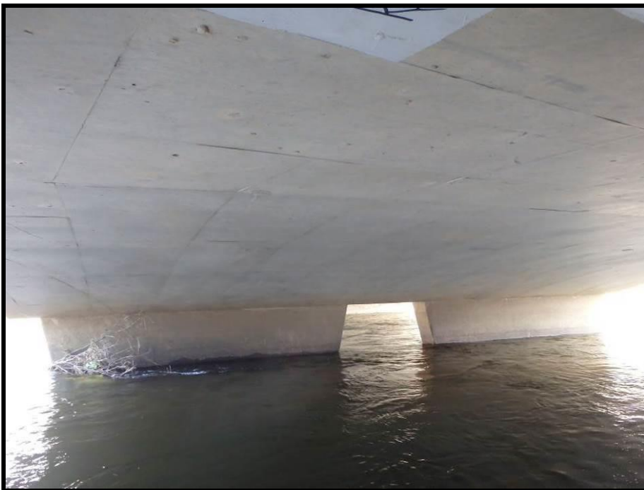
Plate 6 – Underside of the Seamus Rafter Bridge in Enniscorthy town
