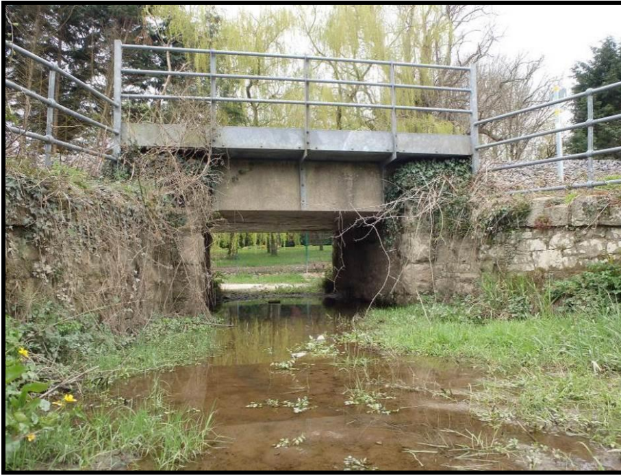
Plate 11 – Railway Bridge in south west of the Survey Area
