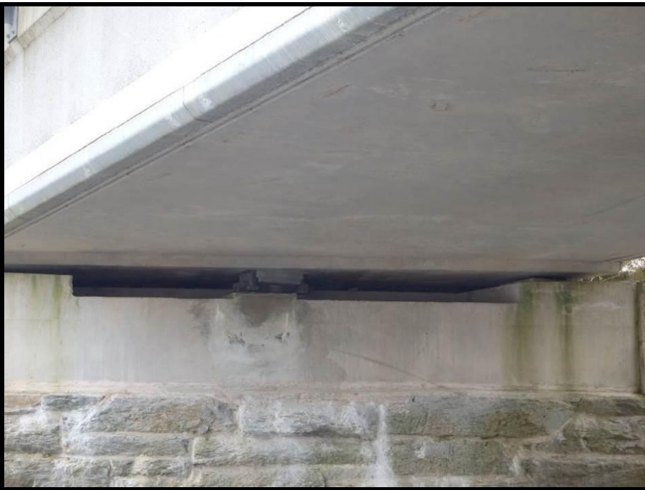
Plate 10 – Railway Bridge over the Urrin River.
