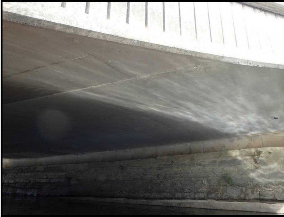
Plate 7 – Abutment joints under the Seamus Rafter Bridge in Enniscorthy
