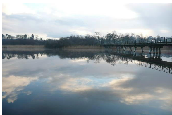
Edermine Bridge at high water
