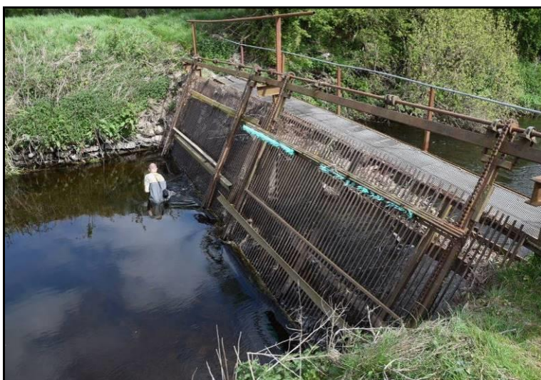
Plate 17: Surveying Clohamon hydro tailrace screen, June 2016. Lampreys and salmonids are entering here and getting trapped below hydro scheme in significant numbers.
