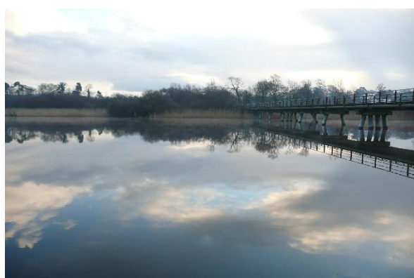
Edermine Bridge at high water
