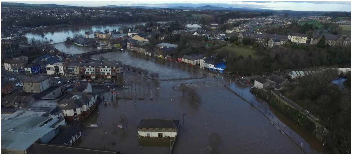
Figure 2: Aerial image of Shannon Quay flooded during 2015 Flood Event
