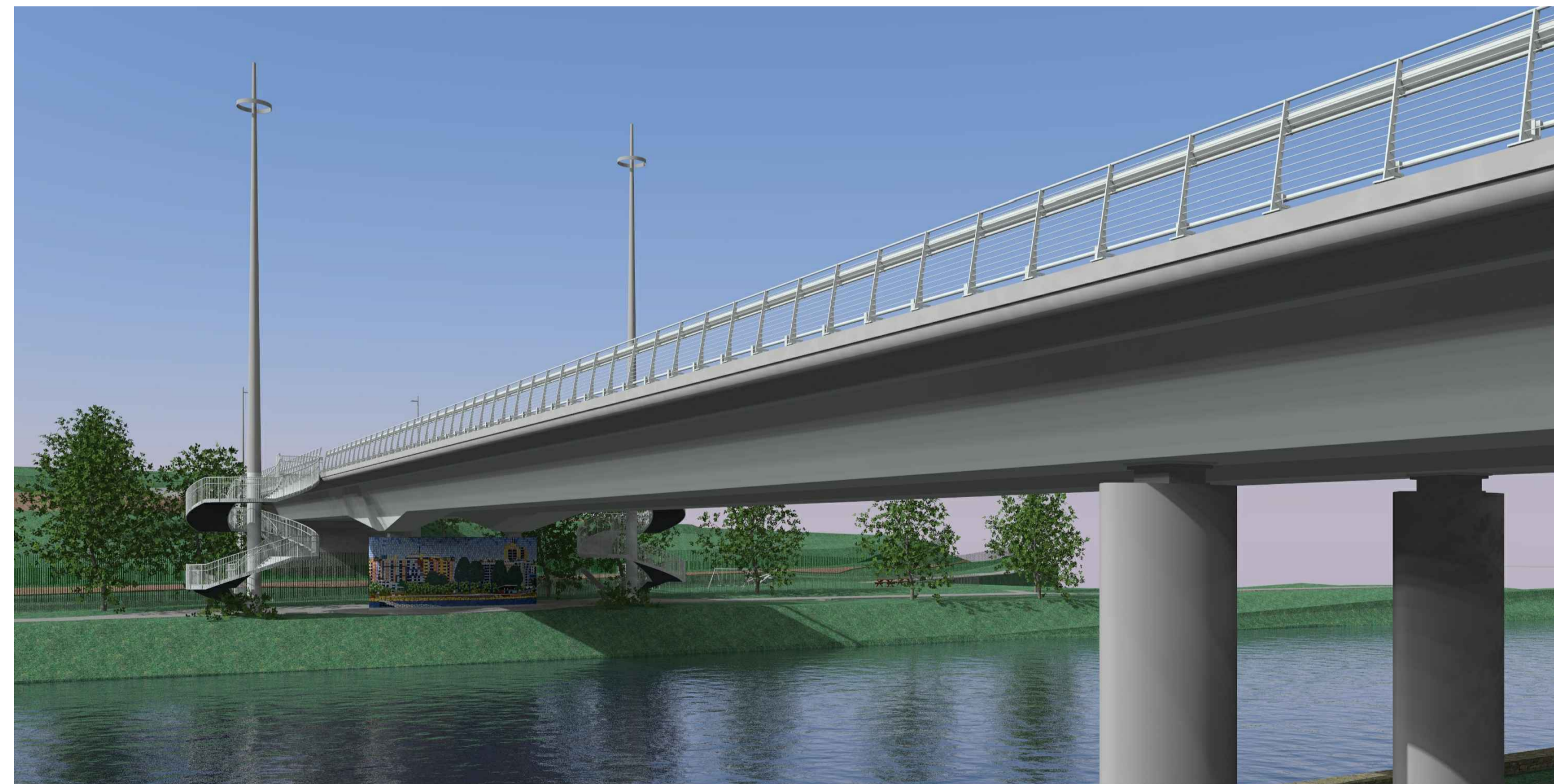
RIVER SLANEY BRIDGE SOUTHERN ELEVATION
